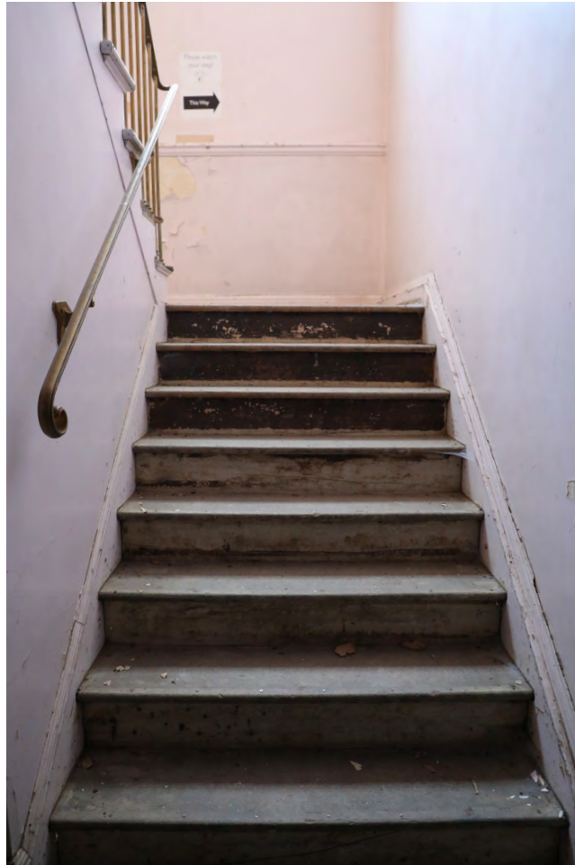
Figure 43 - North stairs from basement, view south (ARG, 2024)
