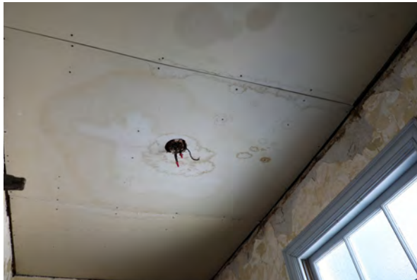
Figure 38: Moisture damage, unfinished drywall, and removed light fixture at ceiling of west Women's Restroom (Room 112)
