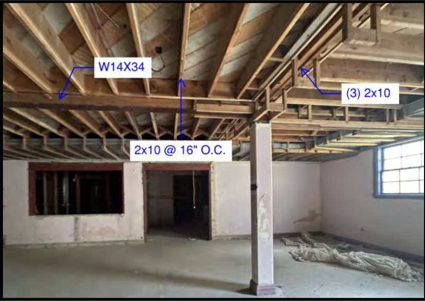
Figure 12 View of the first-floor framing from the basement.
