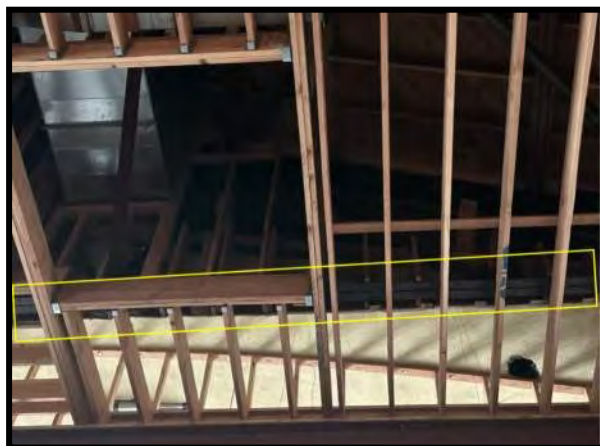
Figure 15 Exposed base of roof truss from Stage.
