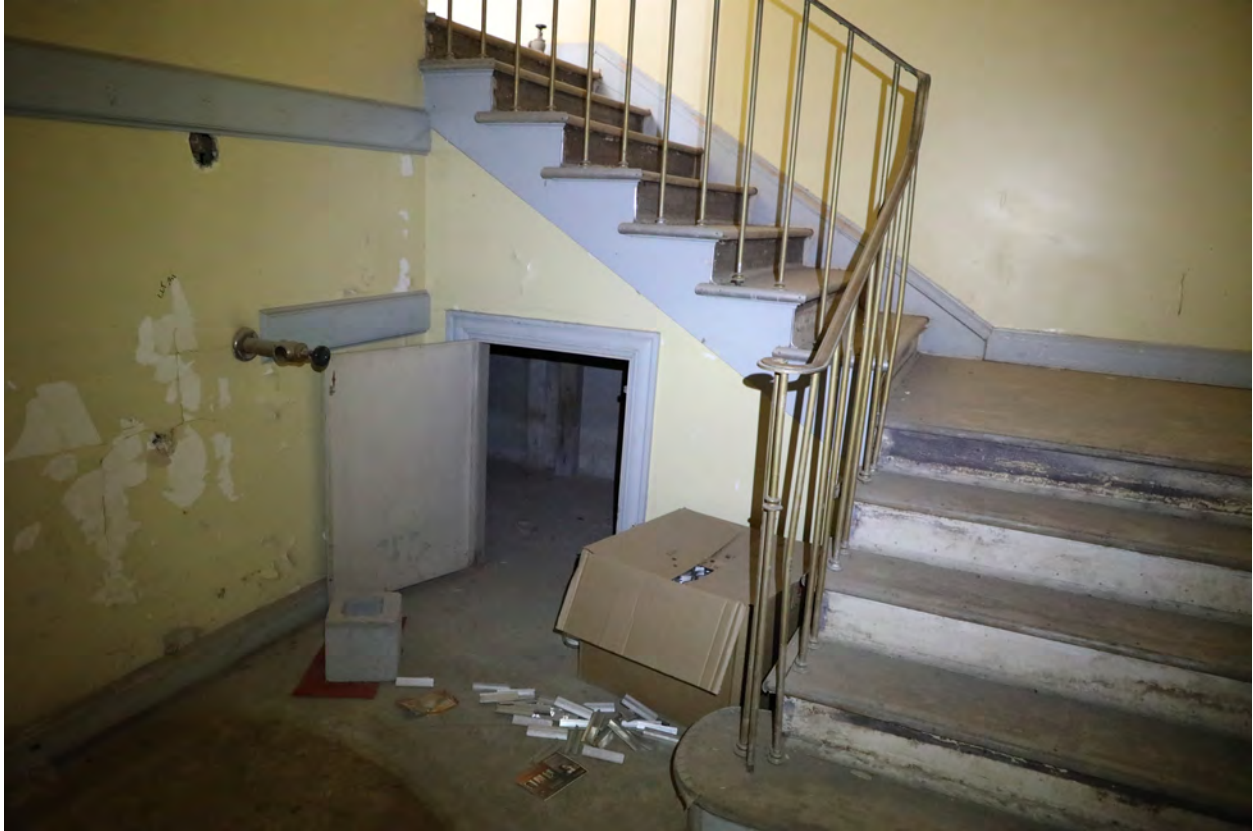
Figure 40 - Basement at base of southern stairs, view southeast (ARG, 2024)
