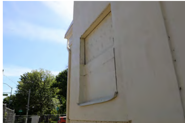
Figure 10: Boarded opening at the east end of the north façade
