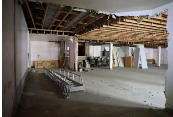
Lear Theater, basement, view northwest (ARG 2024)
