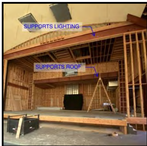
Figure 17 View of steel framing above the stage.
