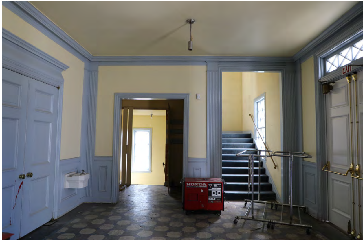
Figure 15 - Foyer, view east (ARG, 2024)
