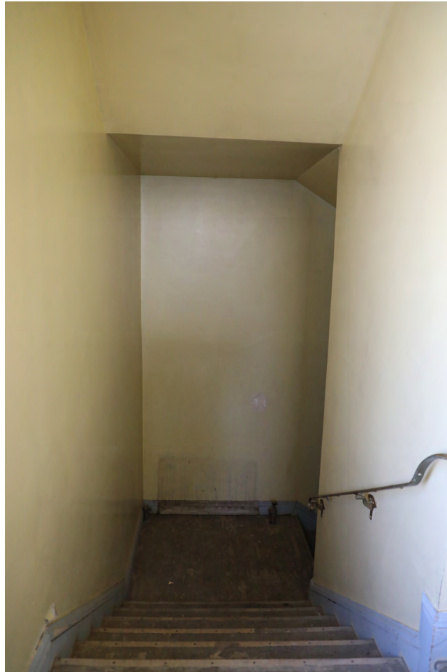
Figure 32 - Southern stairs to basement, view west (ARG, 2024)
