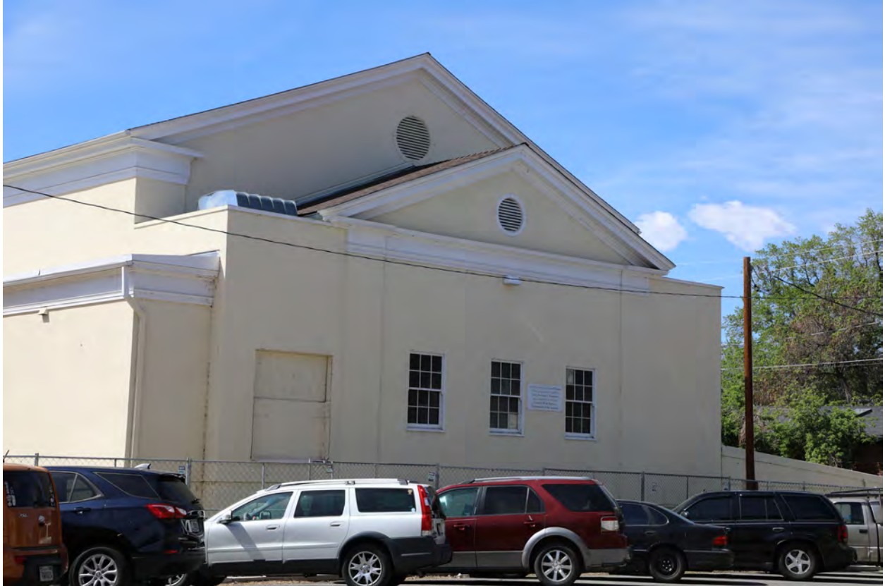
Figure 12 - Rear (north) façade, view southwest (ARG, 2024)
