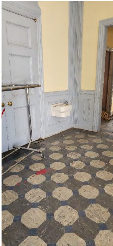
Existing drinking fountain at entry vestibule
