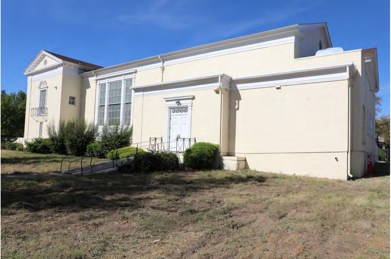
Figure 06 - East façade, view southwest (ARG, 2024)
