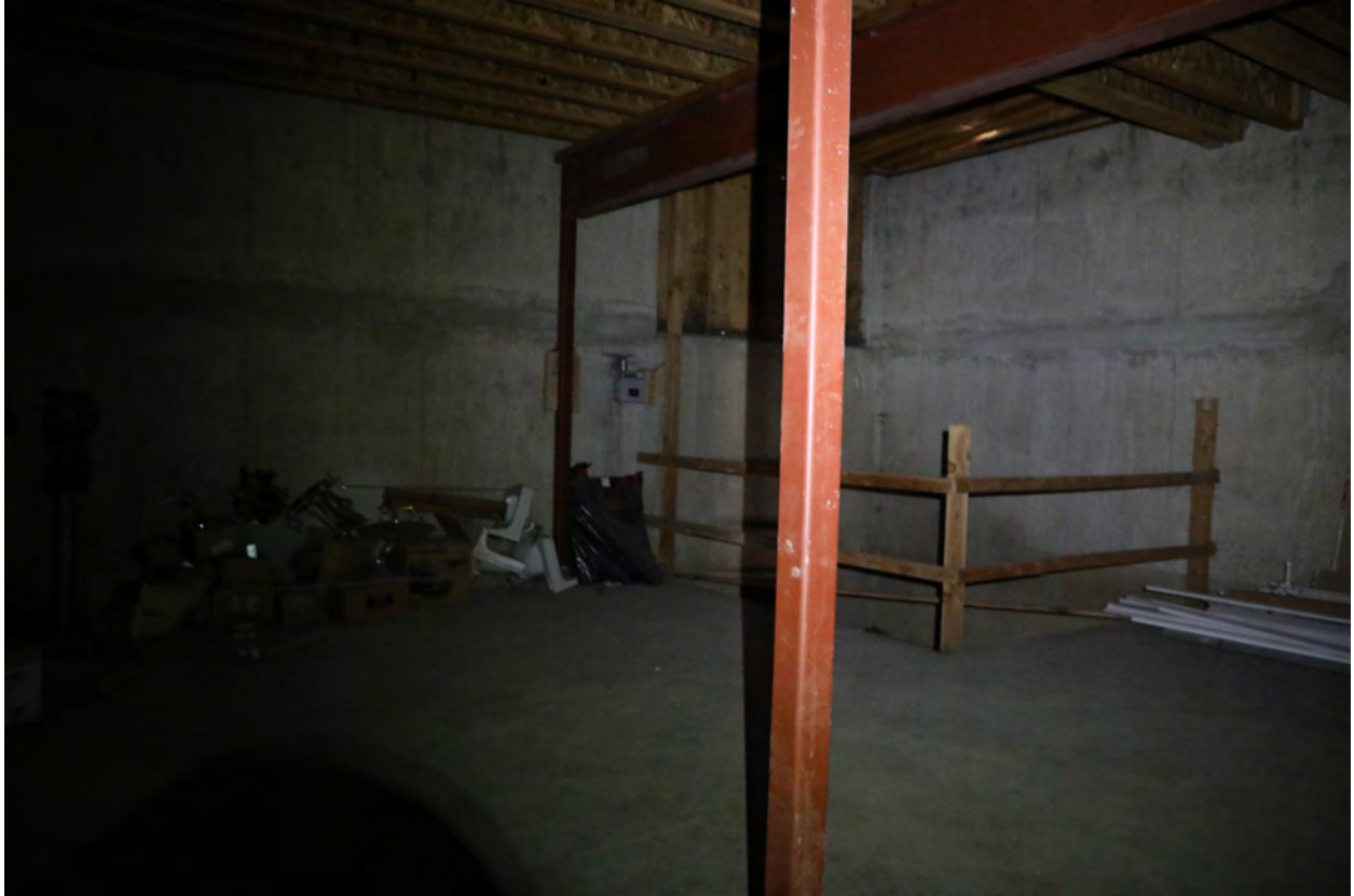
Figure 45 - Basement, looking into unfinished mechanical room with north elevator pit, view northwest (ARG, 2024)
