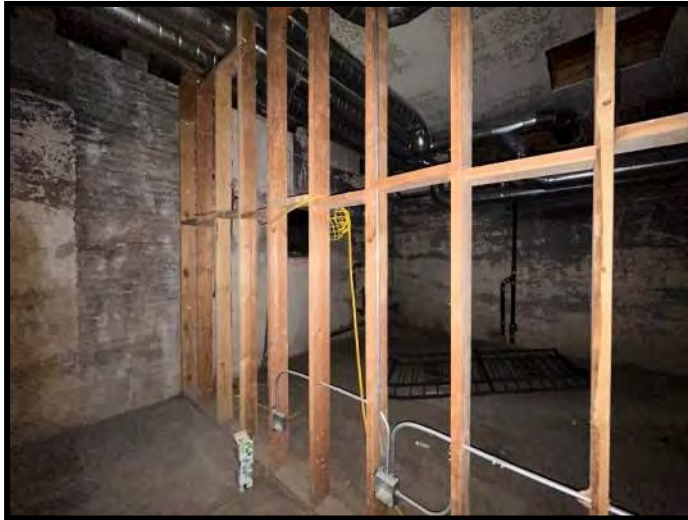
Figure 21 View of an interior wood wall in the basement.
