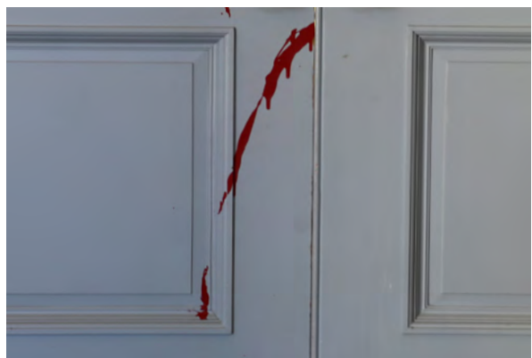
Figure 24: Red paint on Door 1-08 in the Foyer, Room 101
