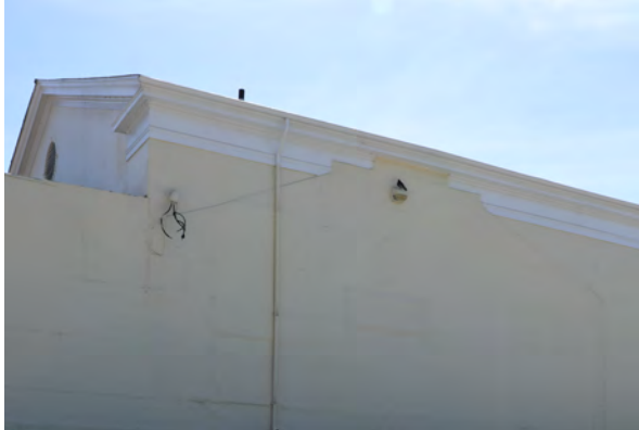
Figure 13: Temporary membrane at the west elevation
