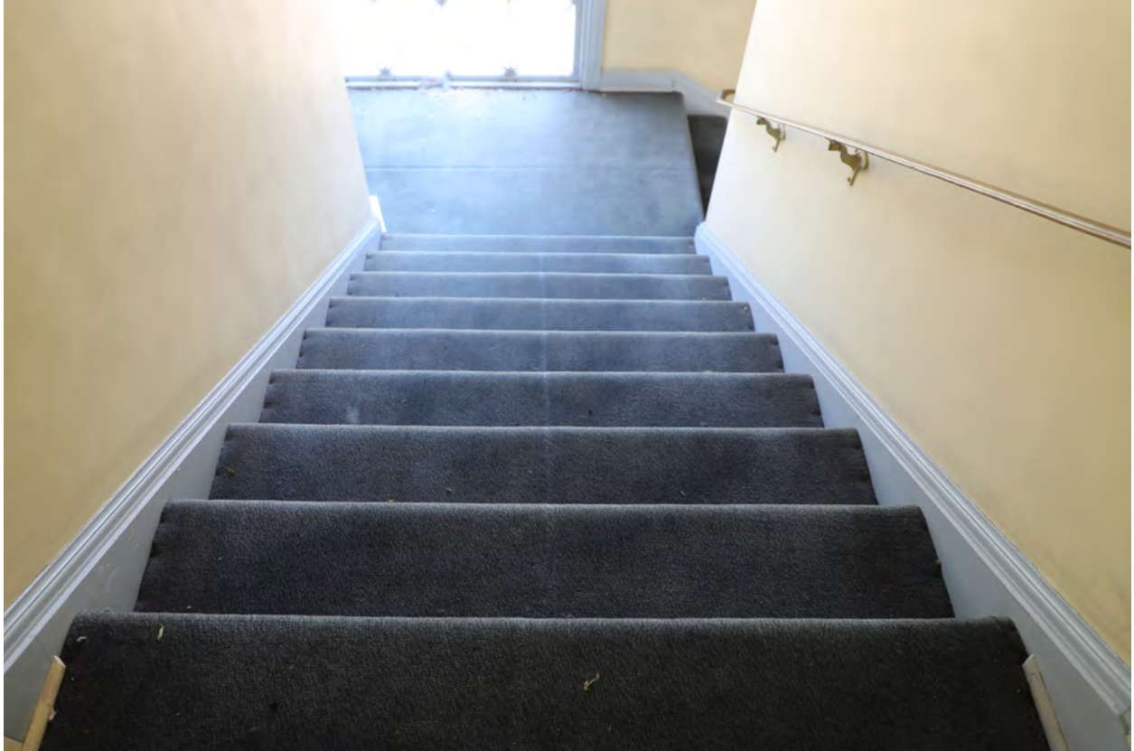
Figure 35 - Stairs to Balcony looking from balcony level, view east (ARG, 2024)
