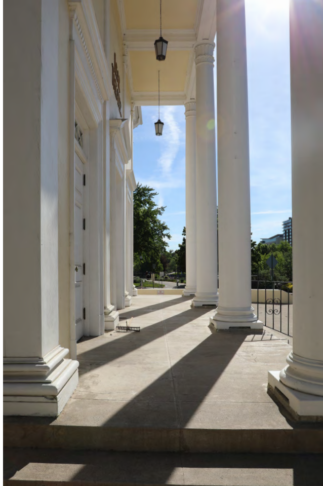
Figure 02 - Porch at primary (south) façade, view east (ARG, 2024)
