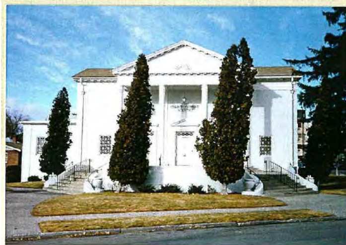
View to the north
