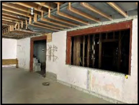
Figure 20 View of an interior concrete wall in the basement from 1938.
