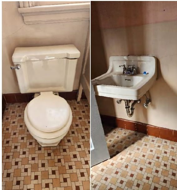
Existing toilet room fixtures:
