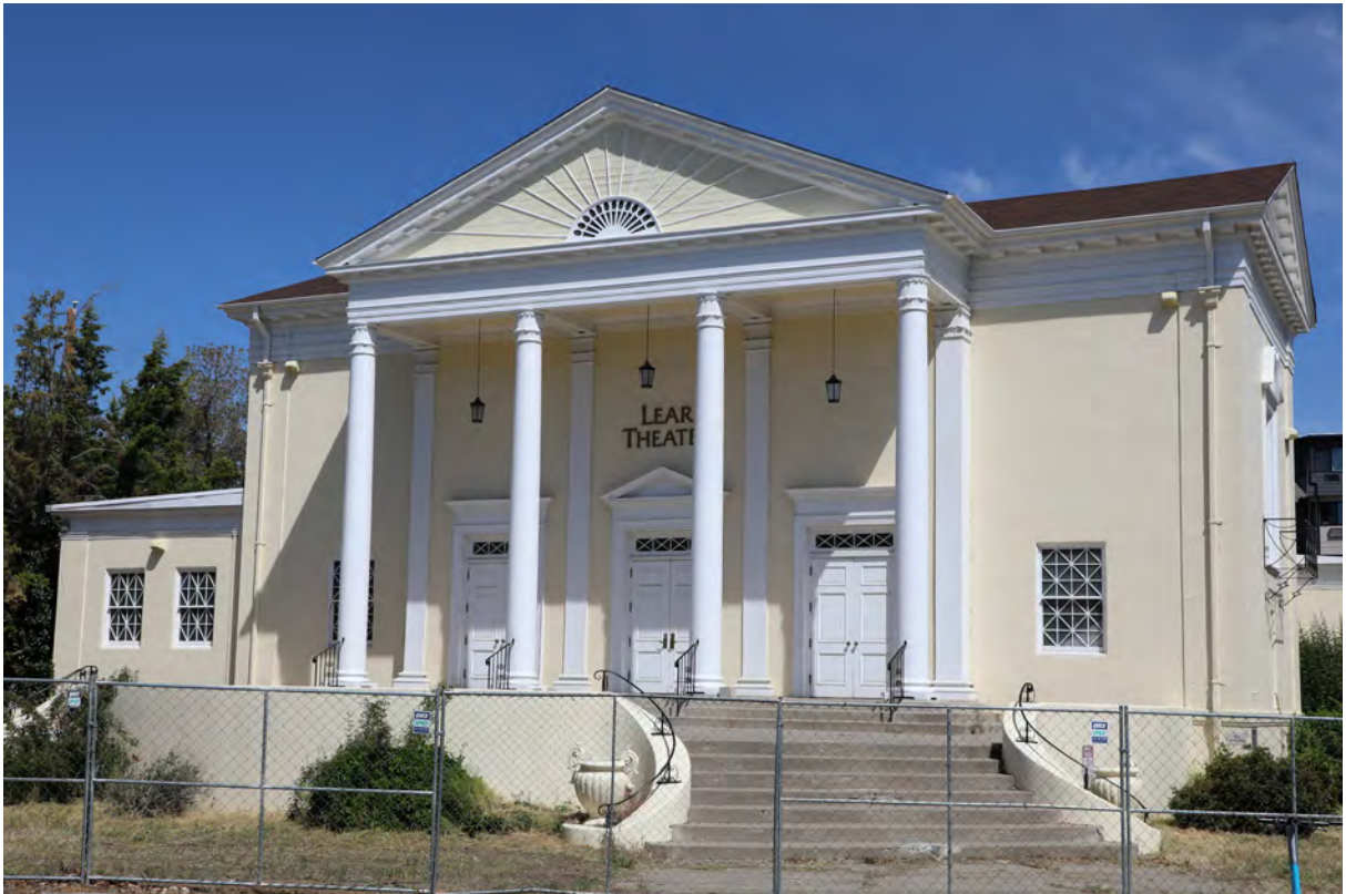
Figure 01 - Lear Theater, primary (south) façade, view north (ARG, 2024)
