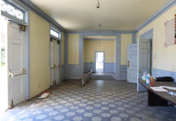
Lear Theater, entry hall, view west (ARG 2024)
