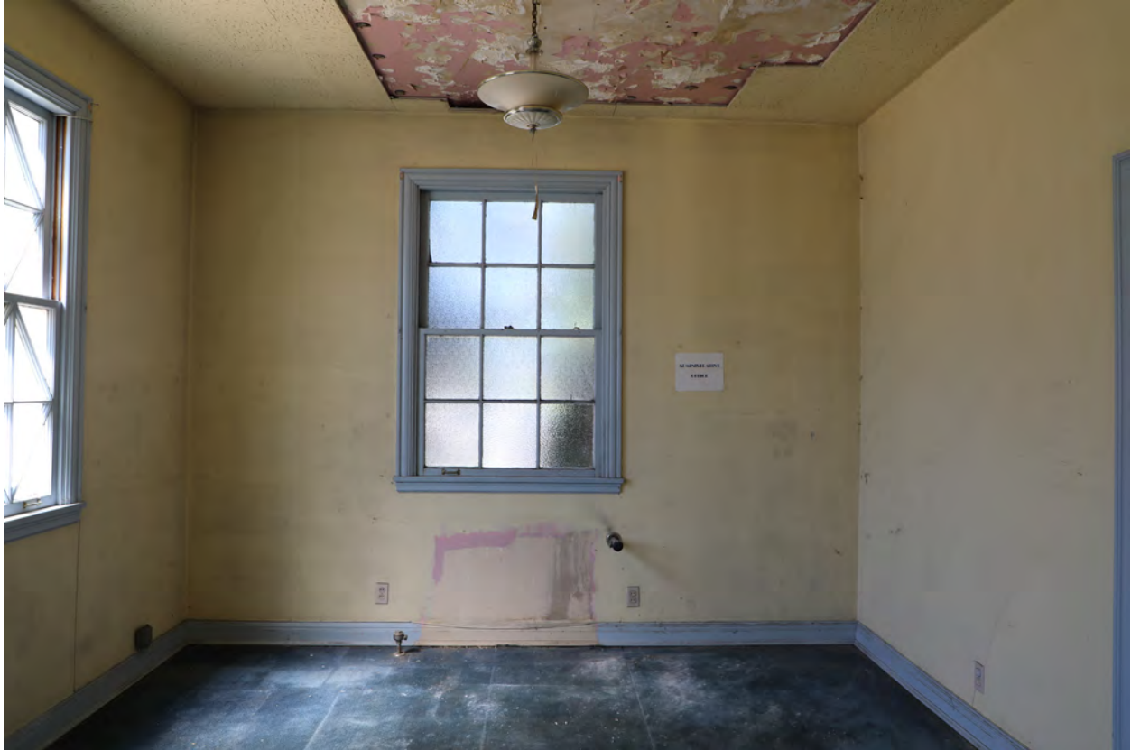
Figure 29 - Literature Room, view west (ARG, 2021)
