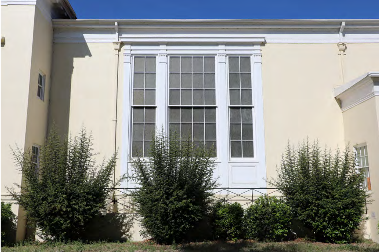
Figure 08 - Central portion of east façade, view west (ARG, 2024)
