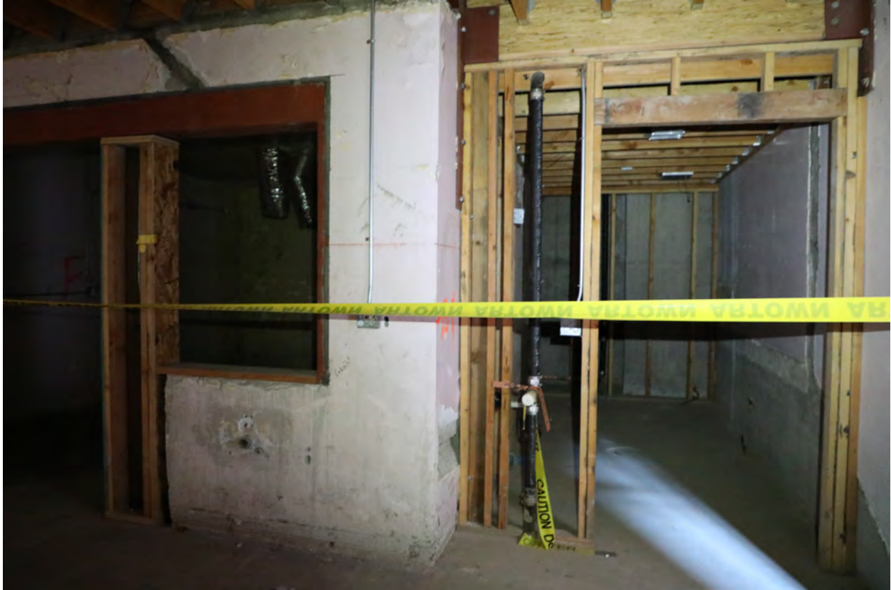
Figure 42 - Basement, northern unfinished spaces, view north (ARG, 2024)
