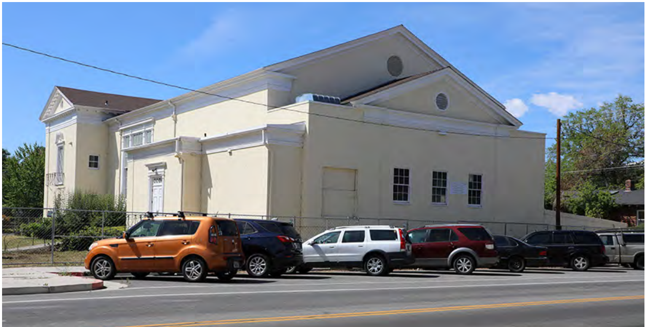
Lear Theater, rear (north) façade, view southwest (ARG 2024)
