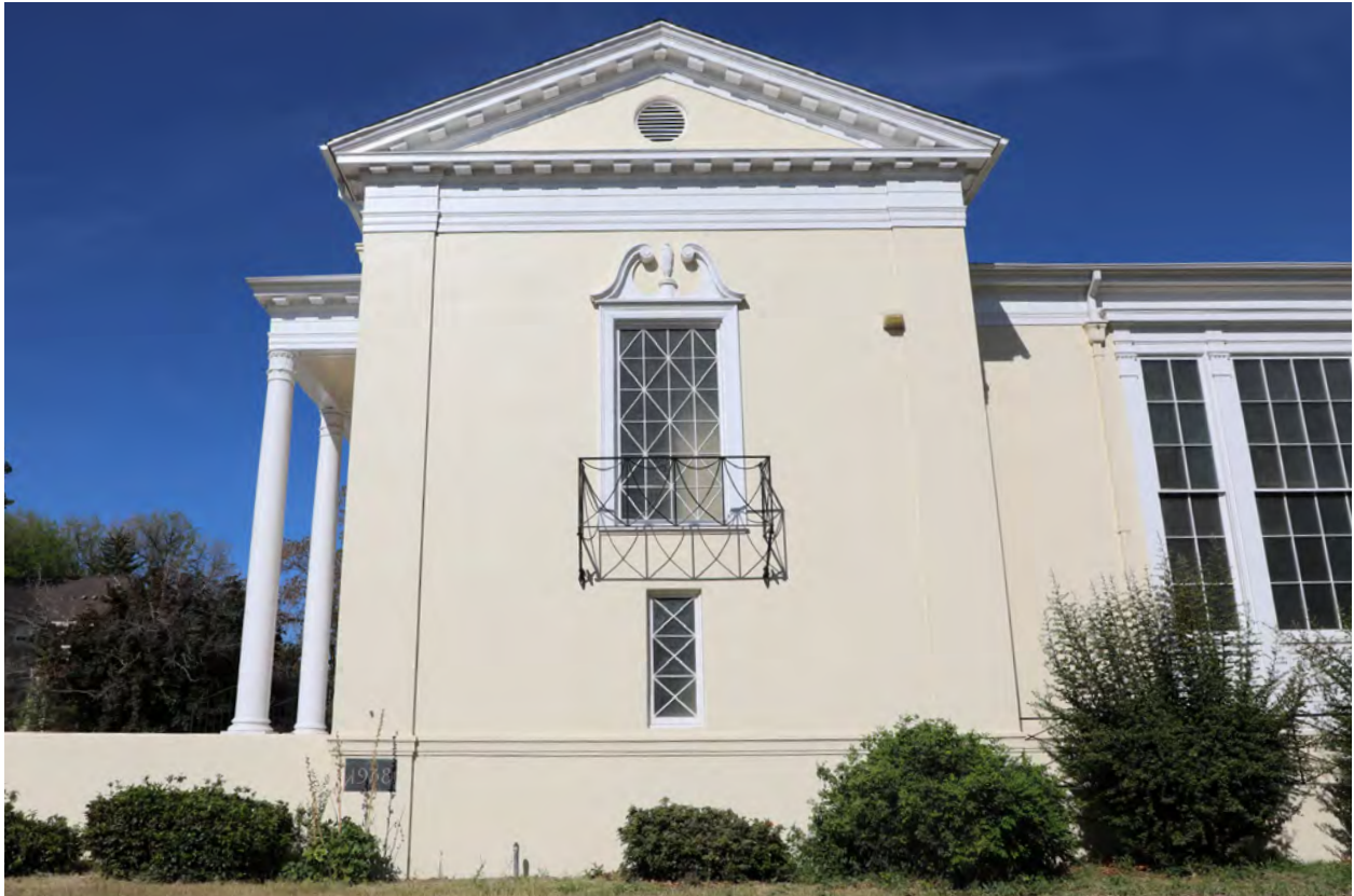
Figure 07 - Southern portion of east façade, view west (ARG, 2024)
