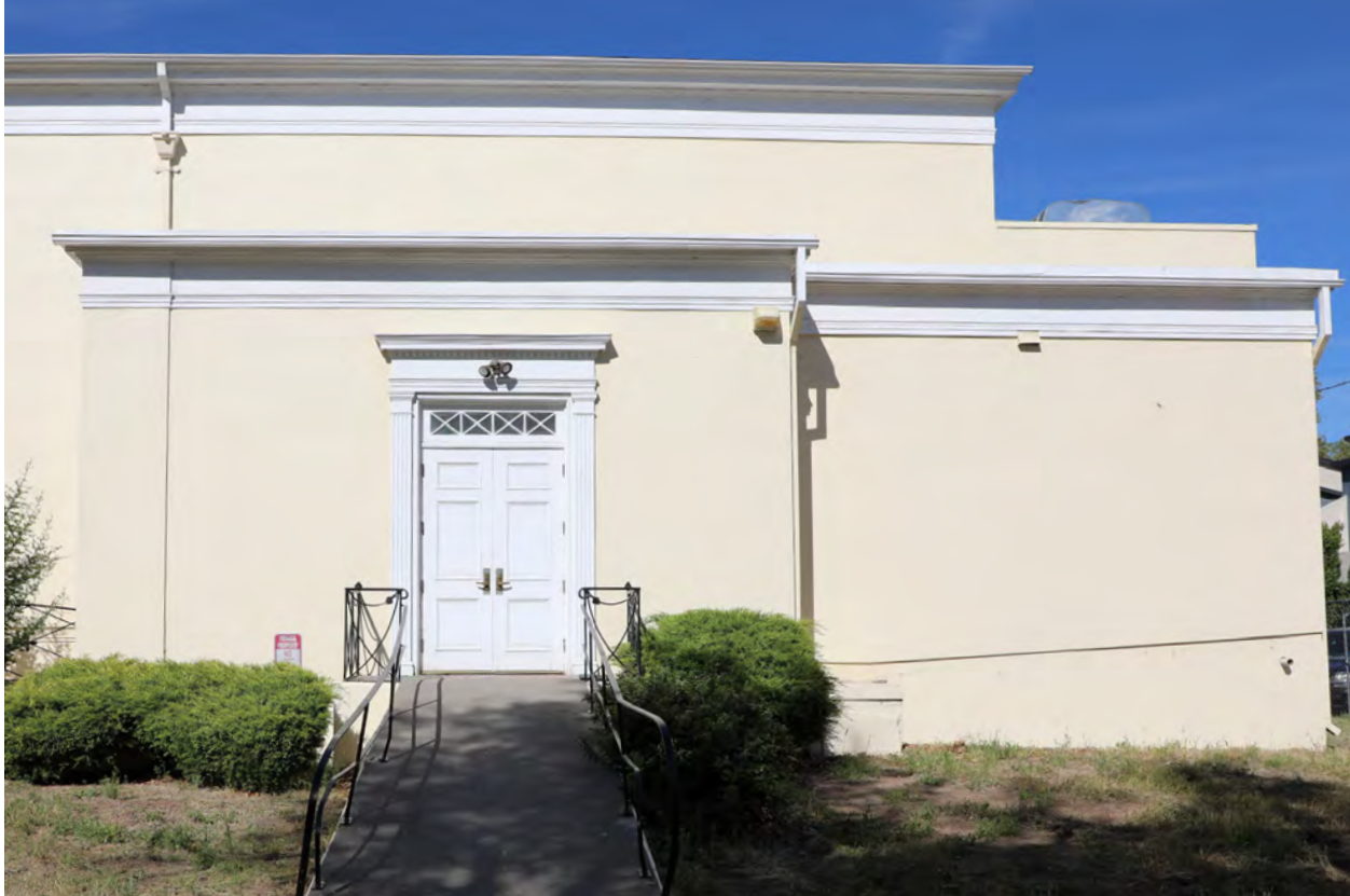
Figure 09 - Northern portion of east façade showing 2002 addition on the right, view west (ARG, 2024)
