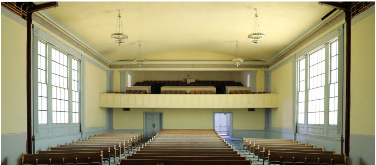
Lear Theater auditorium showing balcony seating area and other original features including pendant light fixtures, multi-pane windows, and decorative painted cornice treatments (ARG 2024)
