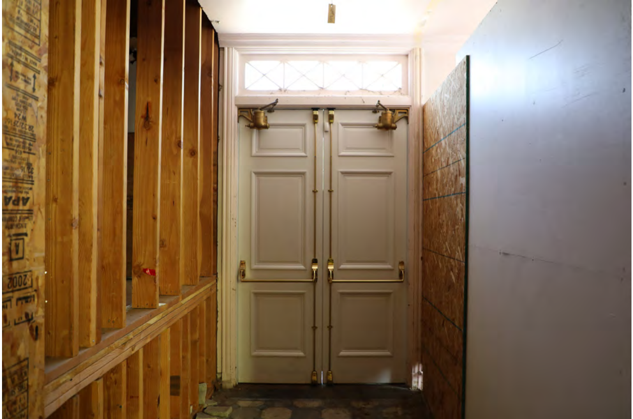
Figure 20 - East entryway, view east (ARG, 2024)
