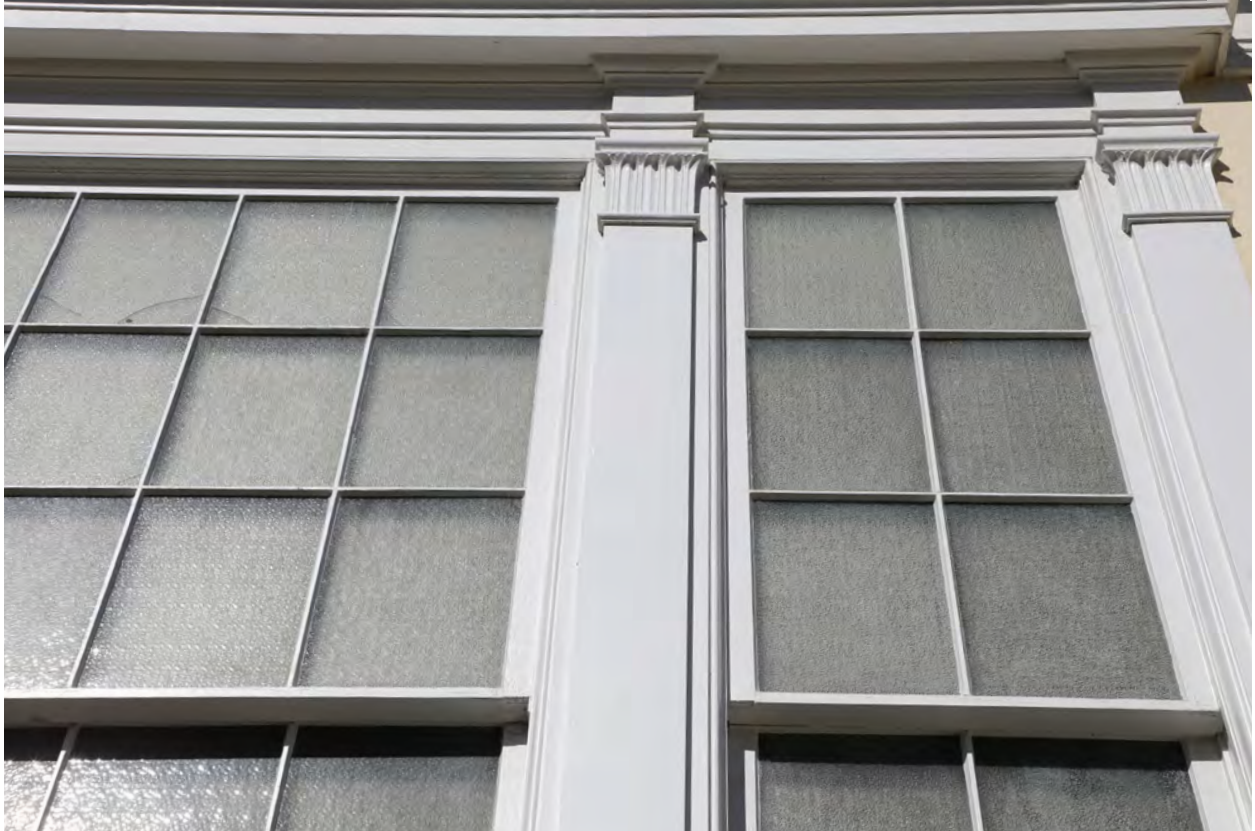
Figure 10 - Detail of large central window at east facade, view west. (ARG, 2024)
