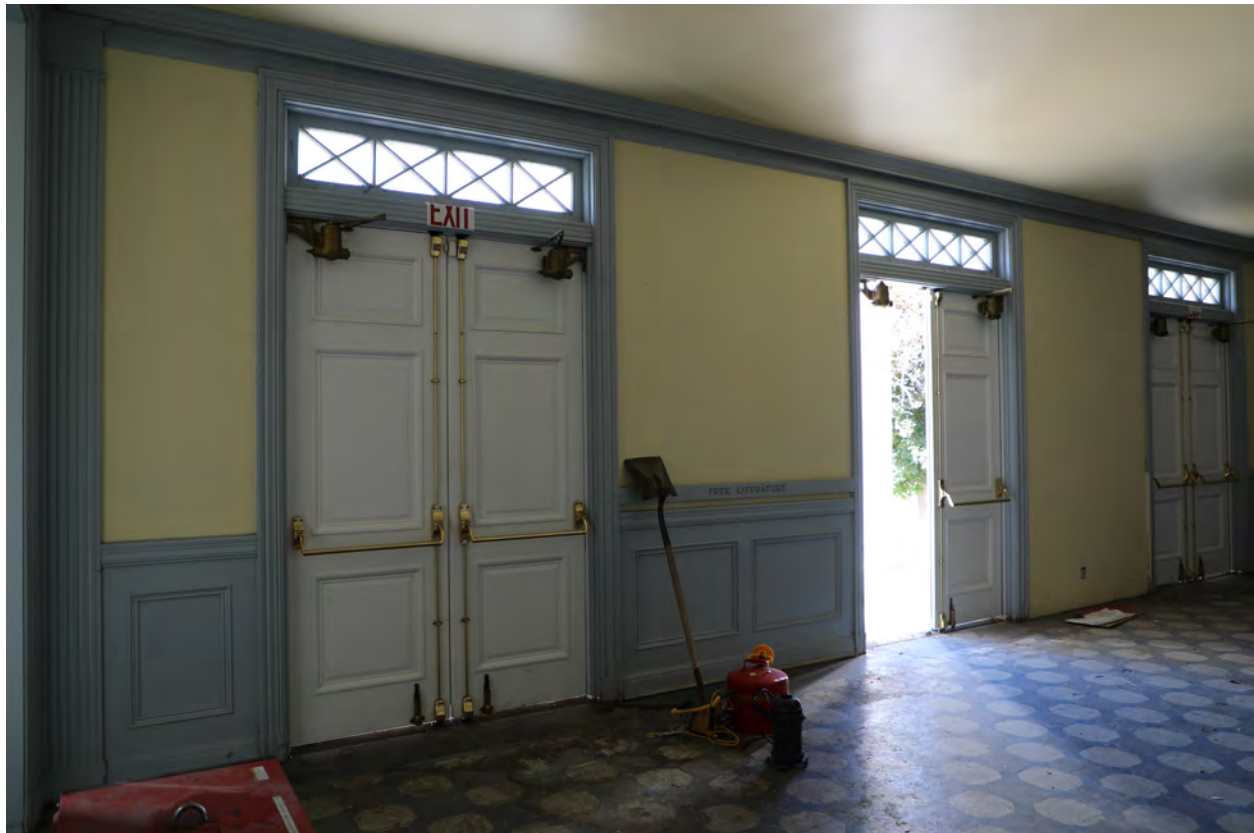
Figure 17 - Foyer, looking toward entry doors, view southwest (ARG, 2024)
