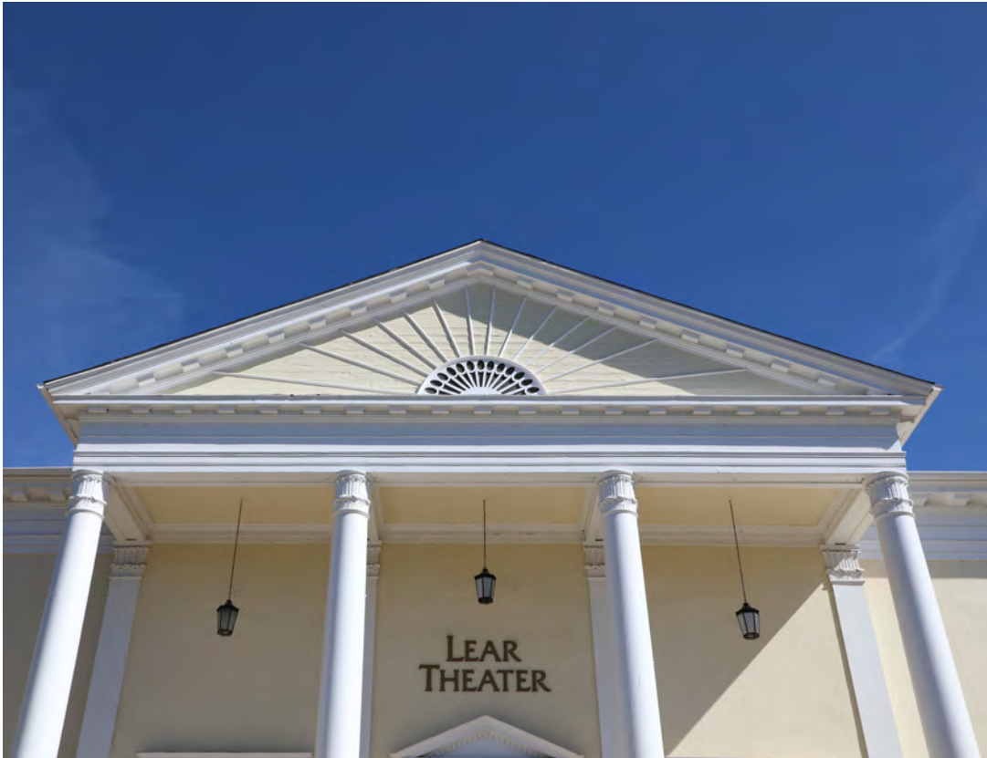
Figure 03 - Gable end at primary (south) façade, view north(ARG, 2024)
