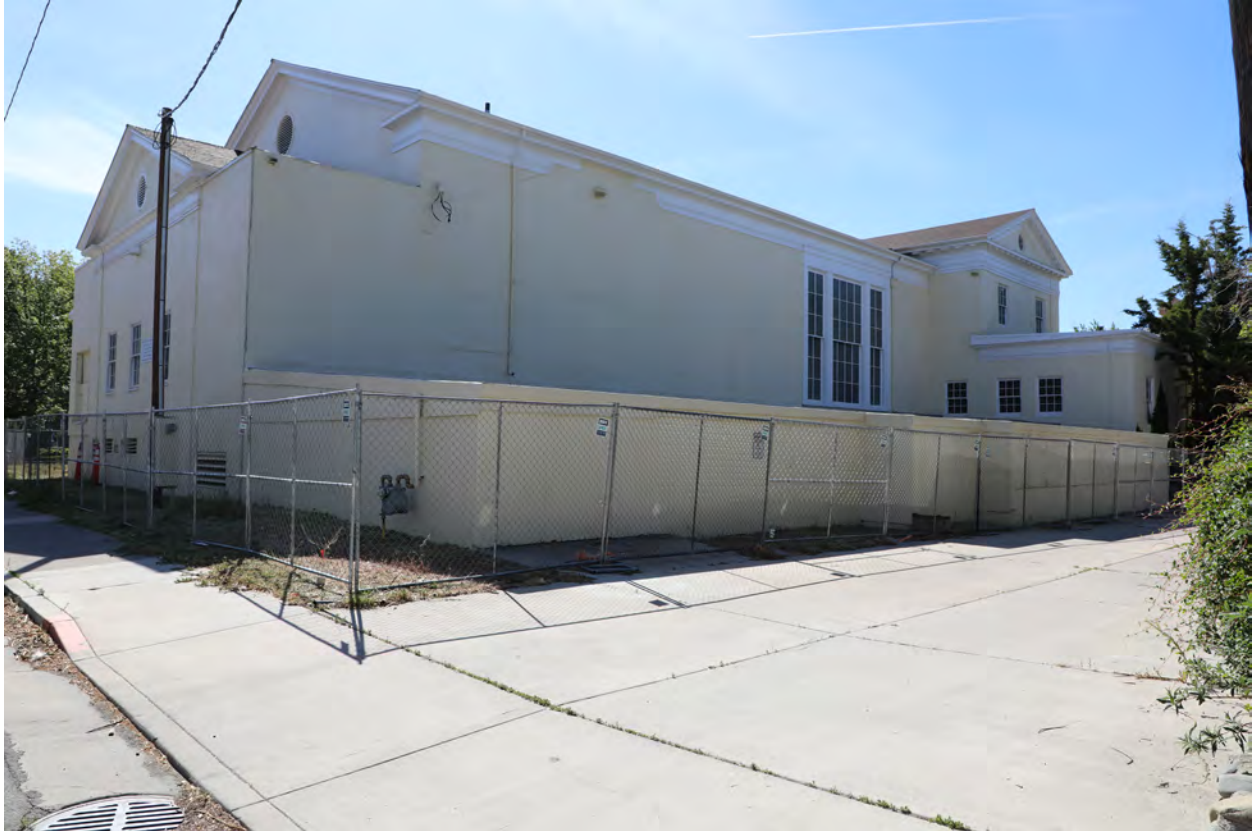
Figure 13 - West facade showing incomplete 2002 addition, view southeast (ARG, 2024)
