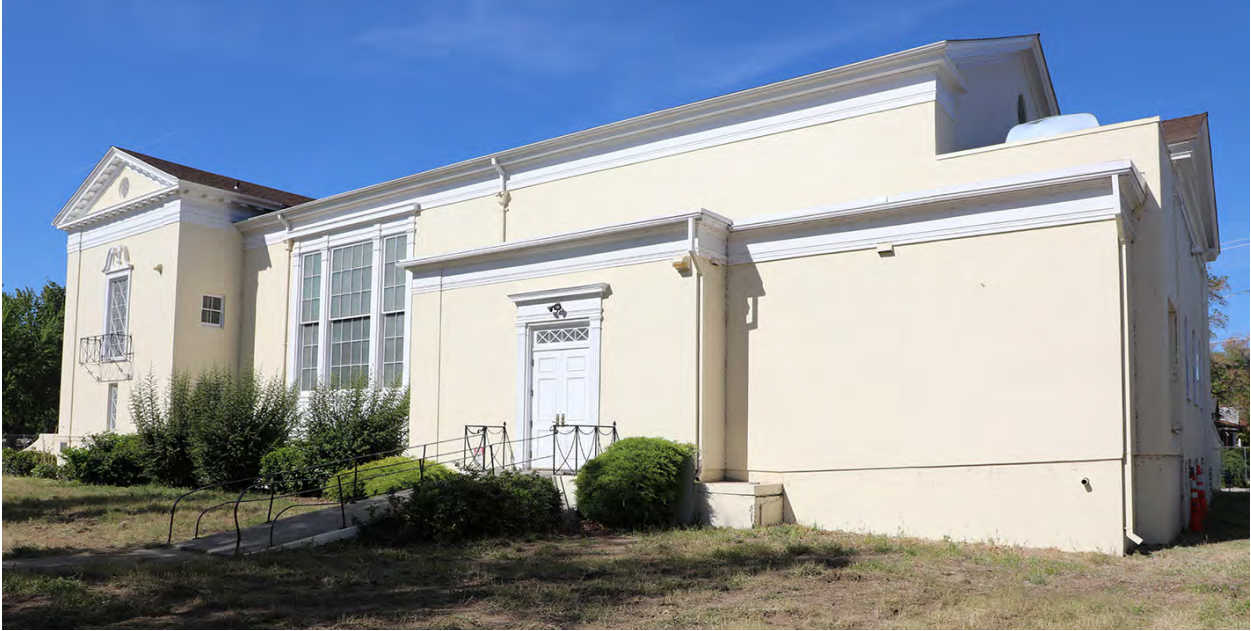
Lear Theater, east façade, view southwest (ARG 2024)
