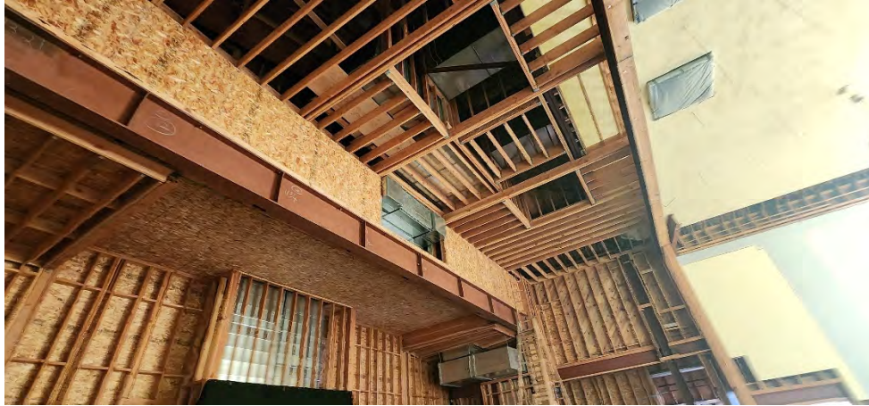
Existing ductwork at existing stage and auditorium ceiling:
