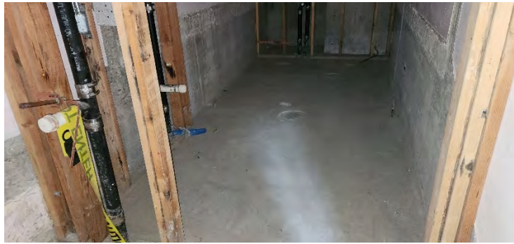
Existing waste and vent system in basement:
