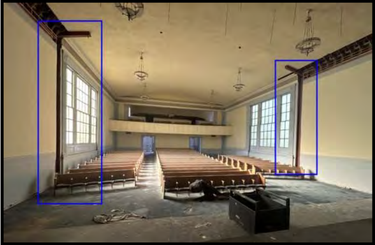
Figure 19 View of the steel TS7x7x1/4 columns from the stage.
